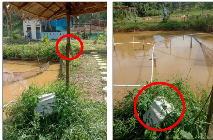
Figure 3. Position of Wooden Pole as Pump Power Source (left side) Figure 4. Fish Breeding Pond and Water Pump Position (right side)
