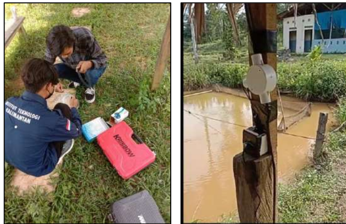
Figure 7. The Aerator Team is Attaching the Hose to the Oxygen Pump (left side) Figure 8. T Boxes and Terminals that have been successfully created (right side)
