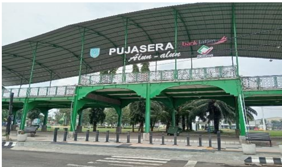
Figure 10. Public Signage at Pujasera, Probolinggo City Square.
