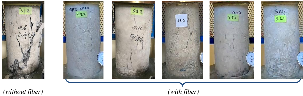
FIGURE 7. Crack after compression test
